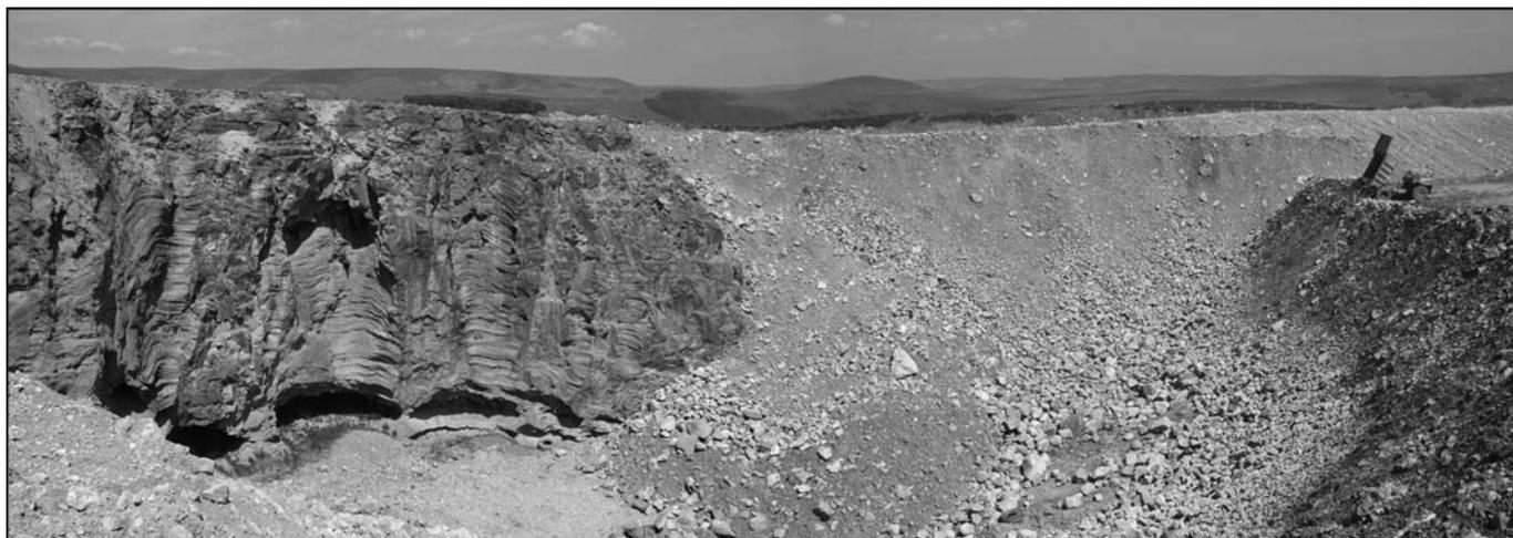
*Backfilling the open pit in summer 2007. The tipper is on the fill at its intended level, which will finally reach a slope down to the foot of the face with the solution features.*
