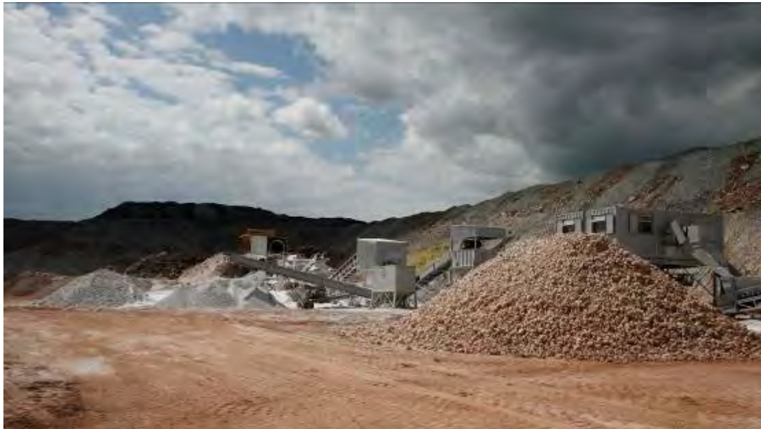
Photo 8: General view of crushing and screening plant. On the far right is the picking shed where hand sorting of lump ore is employed to remove obvious mudstone contamination for the production of best quality white gypsum. Further processing for the manufacture of high-grade gypsum products takes place at the nearby Jericho Works.
