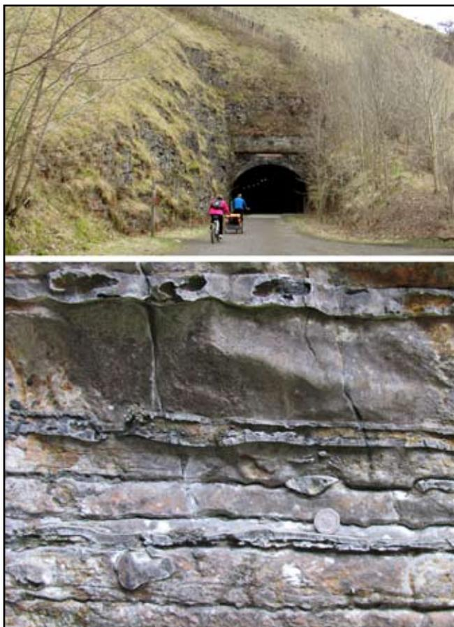
**Figure 5.** Rock cutting at the approach to Cressbrook Tunnel on the Monsal Dale Trail, with a close-up view of the differential face retreat on chert and limestone.
