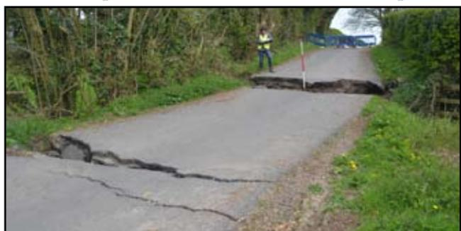
**Figure 6.** Reactivated landslide in Herefordshire (photo: BGS).
