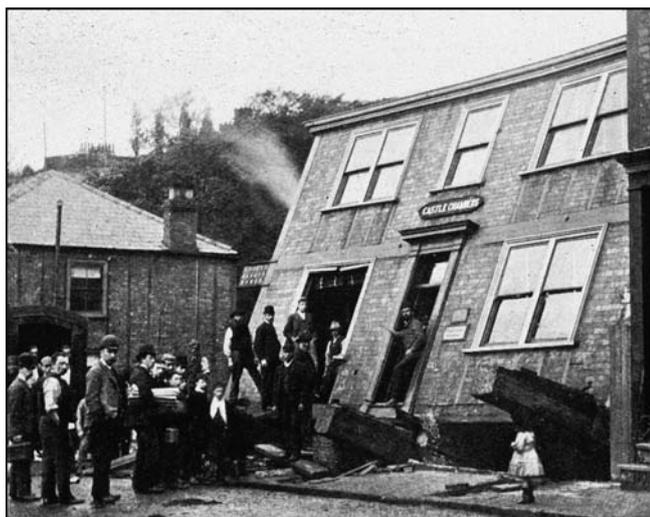
**Figure 1.** Collapsed buildings in Northwich when wild brine pumping was at its zenith a hundred years ago.
