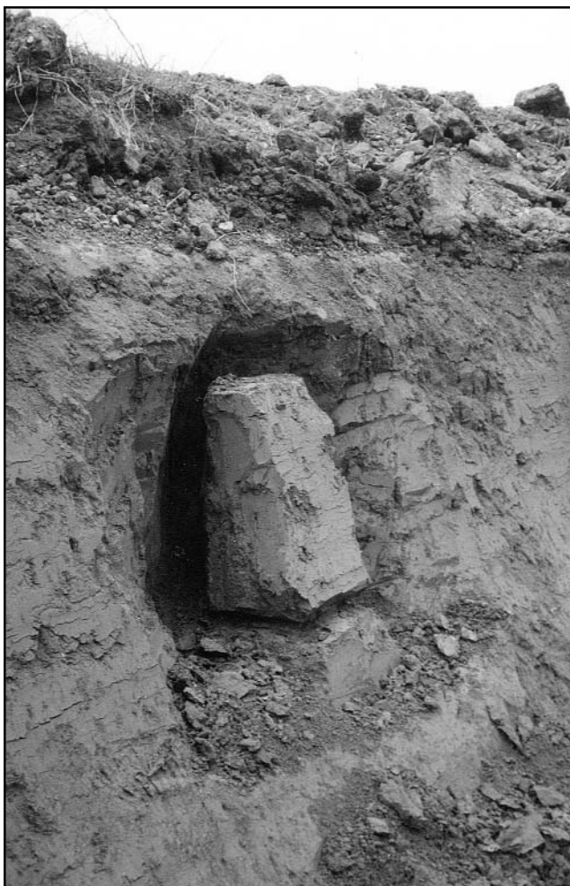
Figure 6. Blocky joints distinguish the weakly cohesive brickearth in a sample 600 mm high from the face of the Ospringe brick pit.
