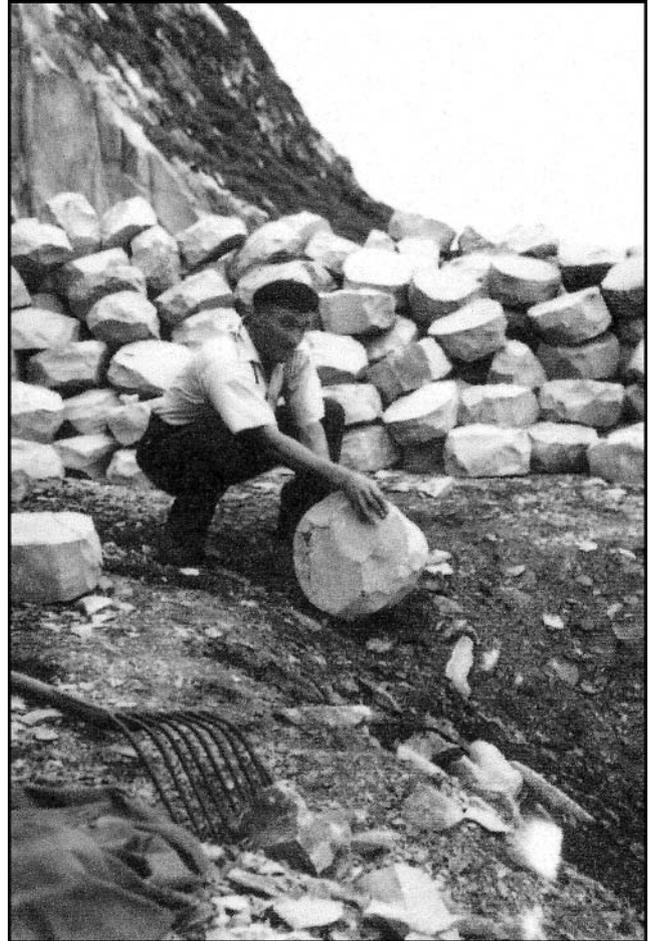
Blocked-out curling stone 'biscuit' being rolled to the foreshore for transport by boat (photograph from BGS Report Vol. 16, No.9, 1987).
