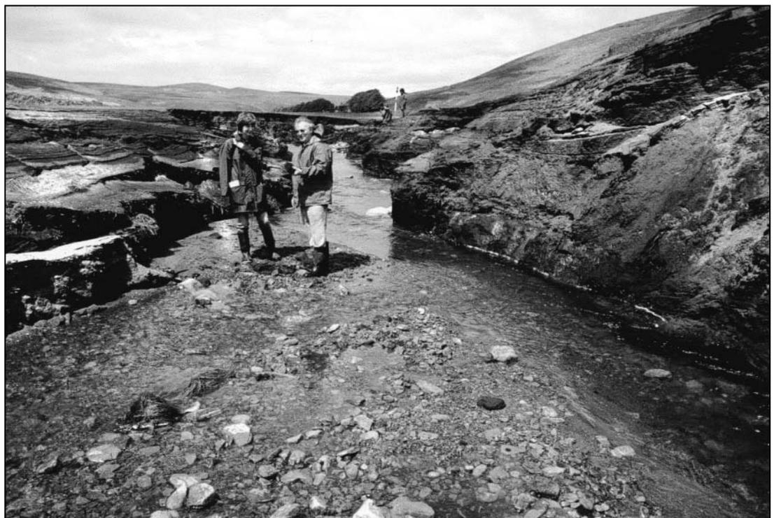
**Figure 7.** Channel cut through sediments in Wessenden Old Reservoir, Yorkshire, when it was drained for repair works.
