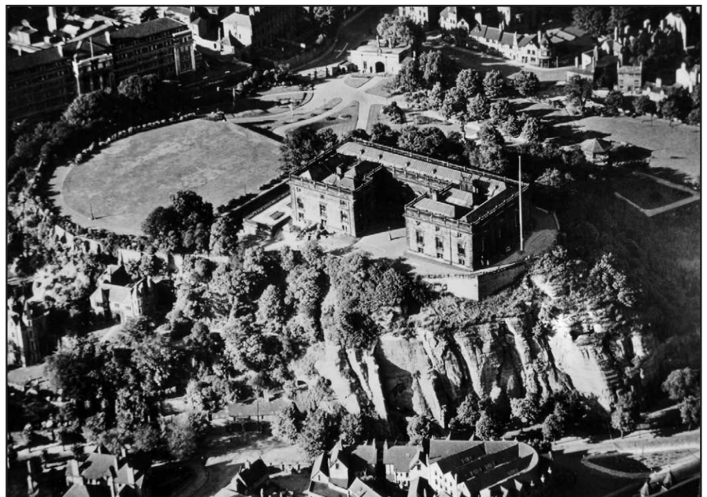
Figure 1. Castle Rock seen from the southwest, with vertical joints defining the serried buttresses of the sandstone cliff.
