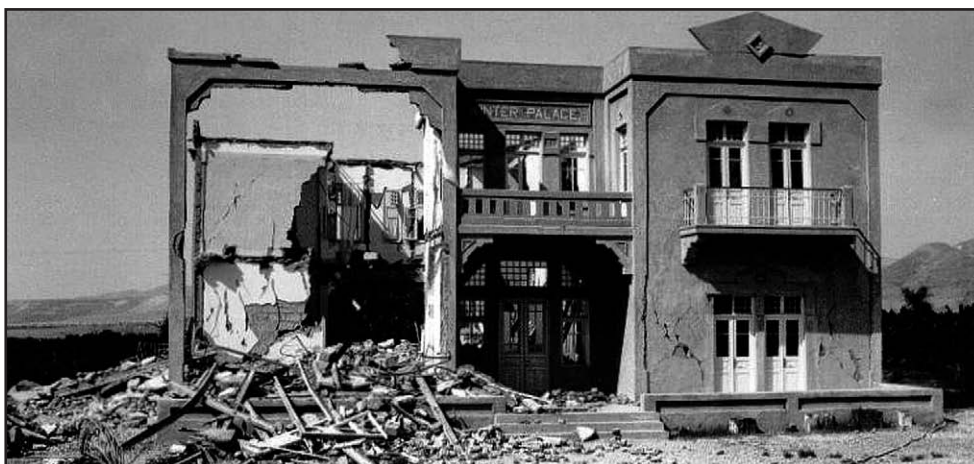
Figure 1. Remains of the Winter Palace Hotel in Jericho, after the 1927 earthquake.
