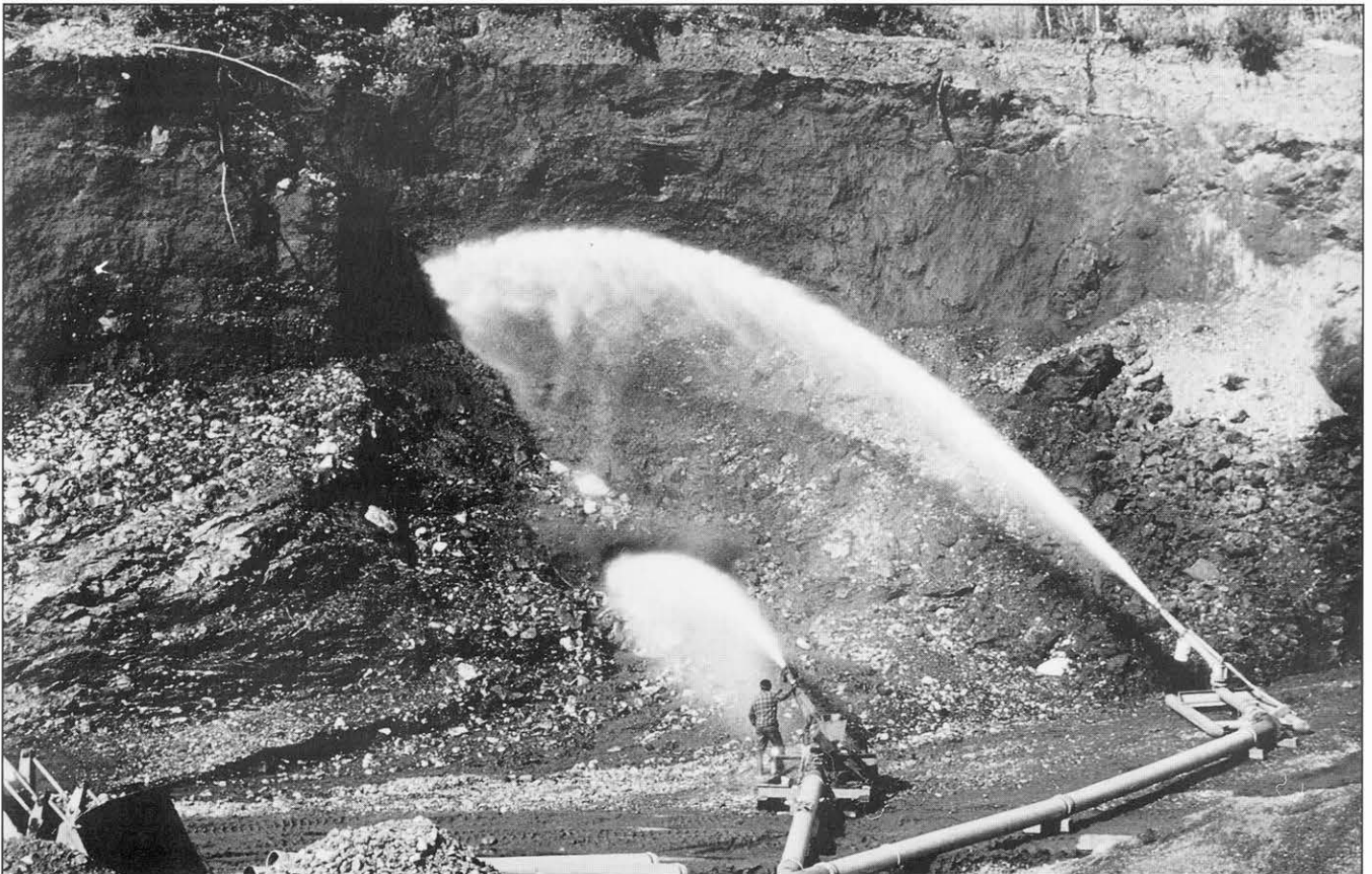
Fig. 7. Monitor pumps in the hydraulicking operation at the Levesque Mine above Hunker Creek. The water jets are cutting into a thick cover of organic muck overlying gold-bearing gravels. Dark Klondike Schist forms the lower half of the bluff to the left of the pumps; its altered and mineralised zone is also being washed out by the water jets. The loose debris is scooped up by a front-end loader and dumped into a sluice off to the left (photo by the author).
