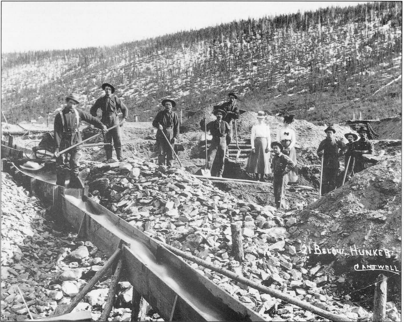
Fig. 6. Early summer on the creeks, with a group of miners shovelling the sediment from a winter's underground digging into their long timber sluice. The photographer's inscription refers to the 21st claim downstream of the first claim on Hunker Creek (photo from the Turnbull Collection held by Dawson City Museum).
